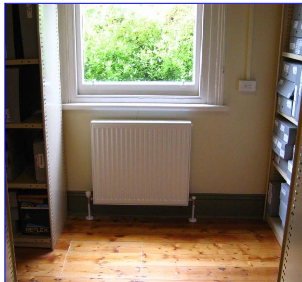
Interior wall panel – Archive room
